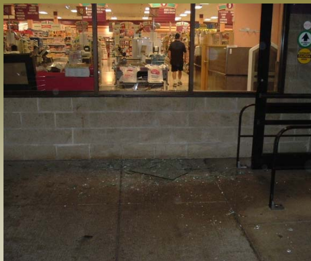
Point of Entry.
